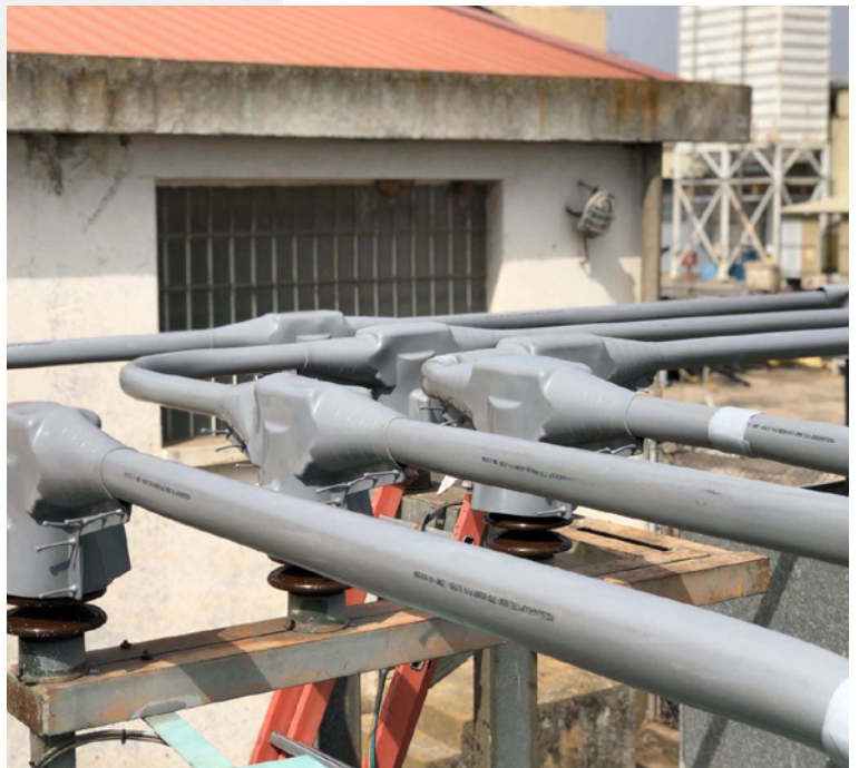
E/Insulation Part # E/INS-200-G being used with E/Bus Support Cover Part # E/BSC
