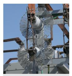
Install E/Flex Barriers vertically on insulator cores to block squirrels, birds, and other wildlife from causing phase-to-ground contact.
