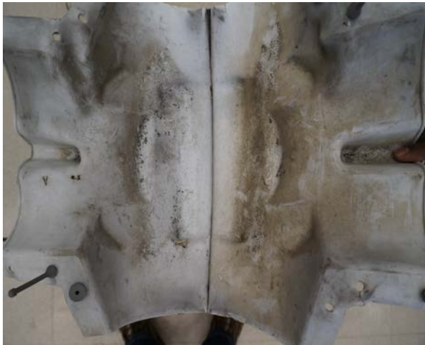
Contamination on inside of E/Bus Support cover.
